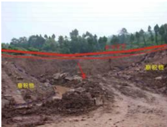
图6. 成都市龙泉驿区某处滑塌体 Figure 6. A landslide-collapse in Longquanyi District of the city of ChengDu.
